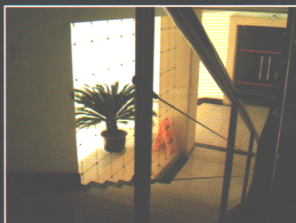
Corporate office stair with 6 mm. angle Slimfix installed
