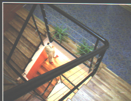
Indoor stair balustrades with 4 mm. angle Slimfix installed
