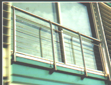
Professional installation of 4 mm. cable balustrades.
